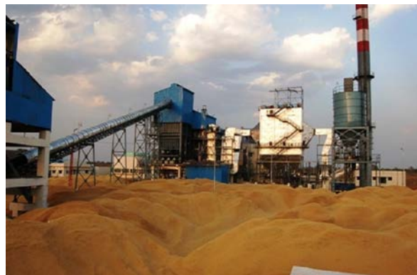
Fig. 1: 10 MW Biomass Power Project
